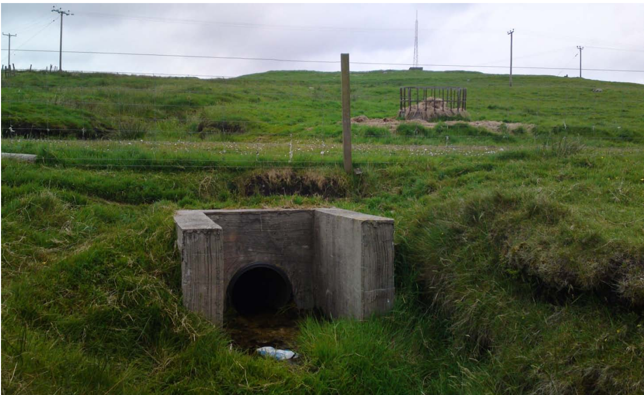
Figure 1.1 Existing drainage infrastructure
