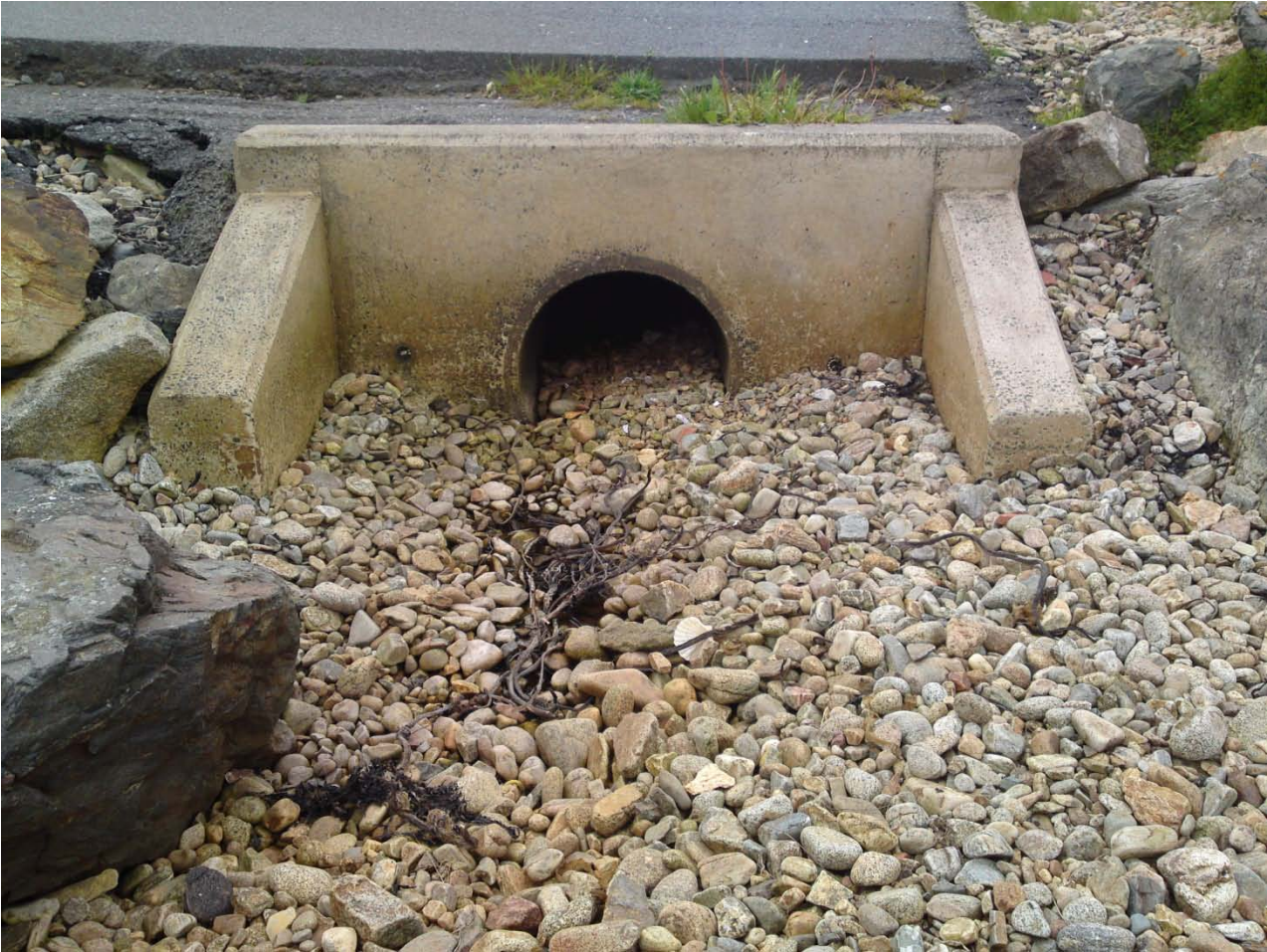
Figure 1.2 580mm internal diameter piped outlet
