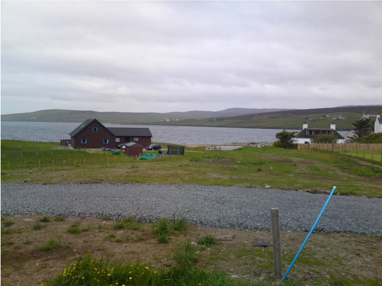
Figure 1: Site looking north
