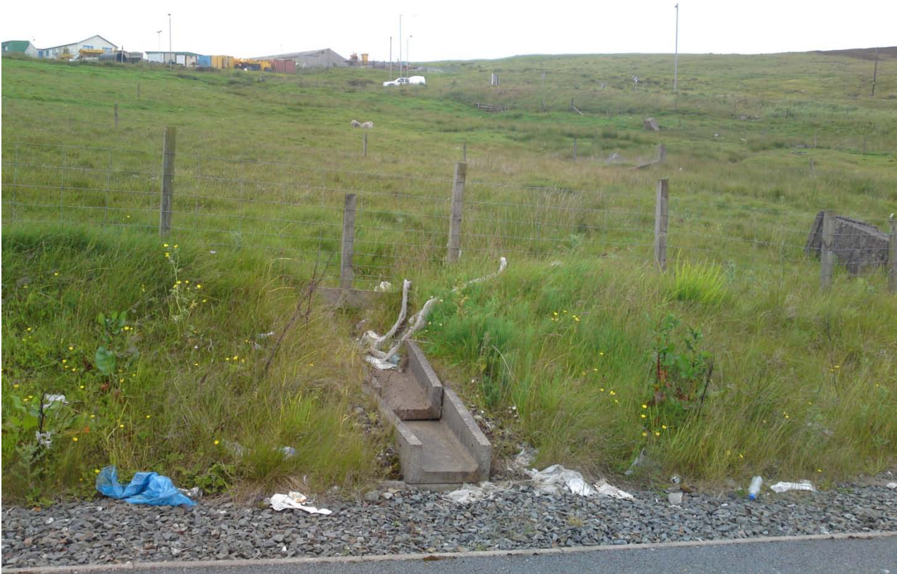
Figure 1.1 Chute drain
