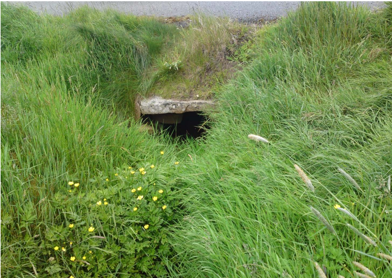
Figure 1.1 Stone Built inlets
