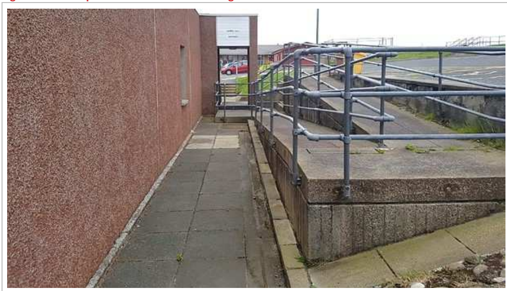
Figure 3.11 Ramped Pedestrian Route Through Site
