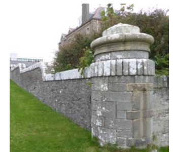
Existing Historic Walls
