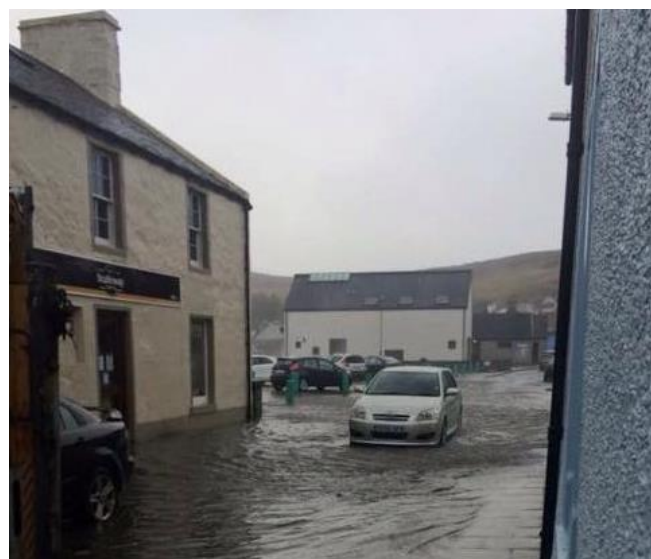
Recent Flooding on Main Street
