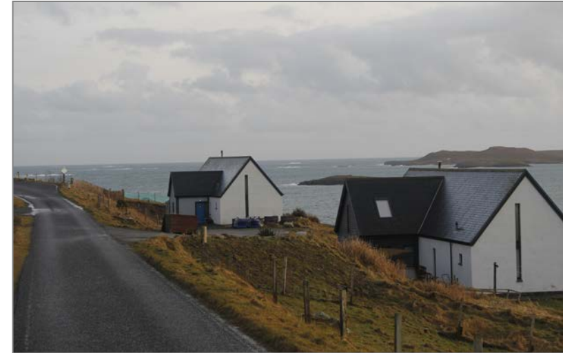
Image 8. Shared accesses within a rural context, can reduce vehicle entry points onto the public road
