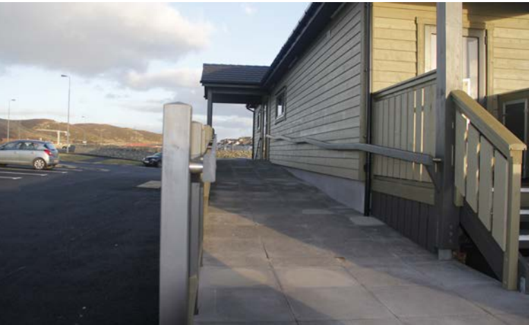
Image 17. Ramps allow for all users of a building
