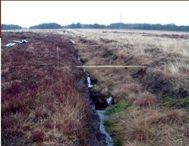
Terminal drain before
