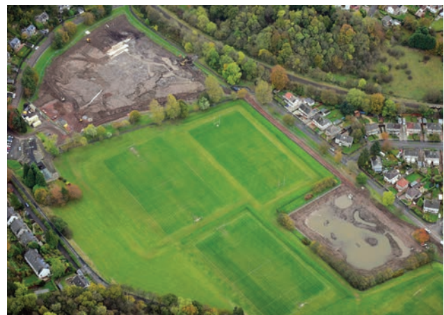
Work in progress: Construction of pond and wetland area, 2014
