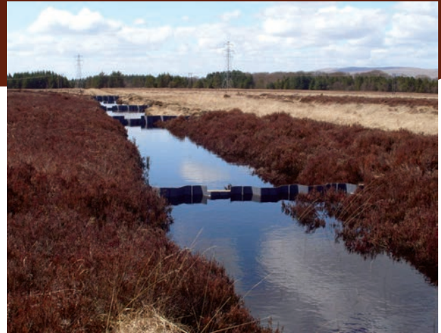
Terminal drain after
