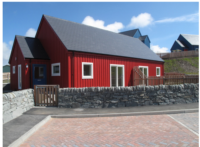
New houses at Burnbank, Lerwick
