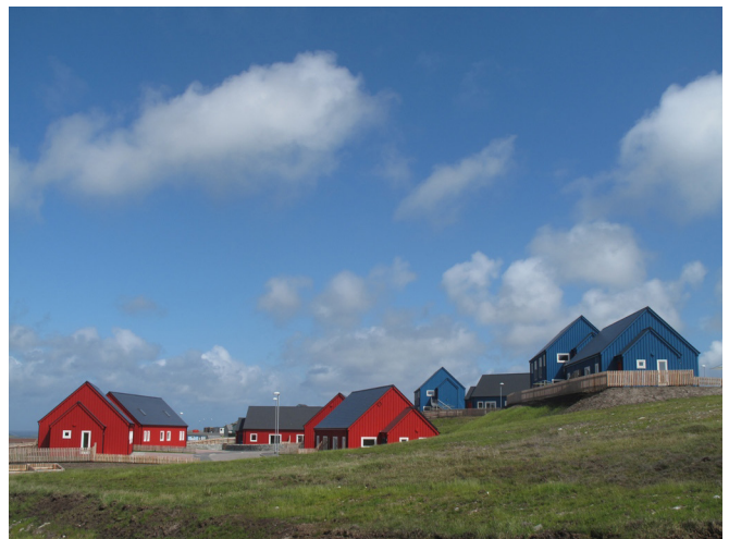
New houses at Burnbank, Lerwick
