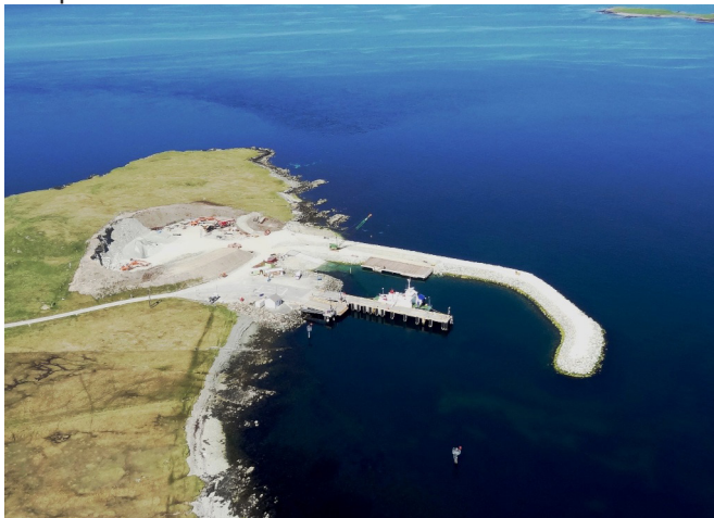
Aerial view of Fetlar Pier
