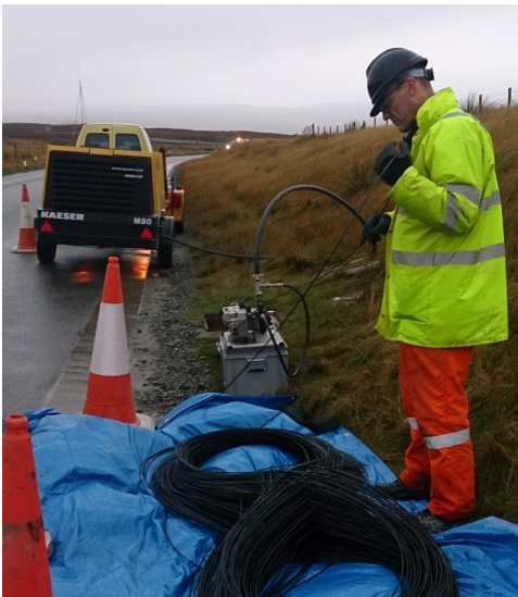
Installing the fibre-optic broadband connection
