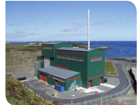
Energy Recovery Plant
