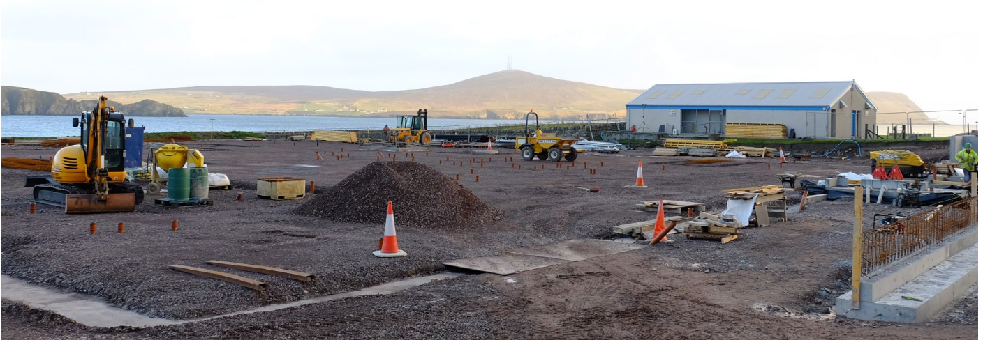
Early work on site
