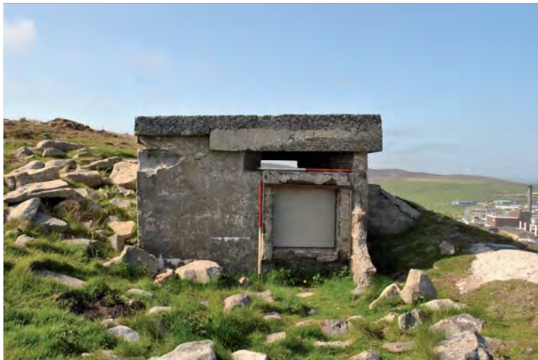
Plate 24: Site 29, south facing elevation
