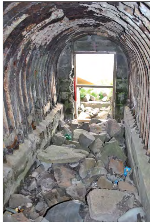
Plate 19: Interior of Site 30 south entrance
