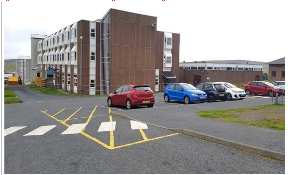
Figure 3.8 Internal Car Park behind High School Buildings
