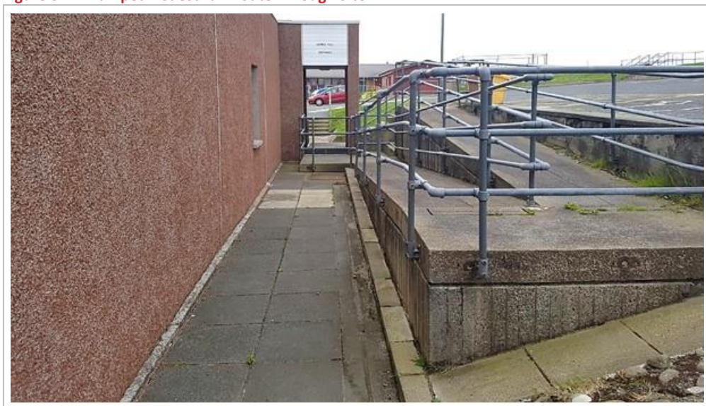
Figure 3.11 Ramped Pedestrian Route Through Site
