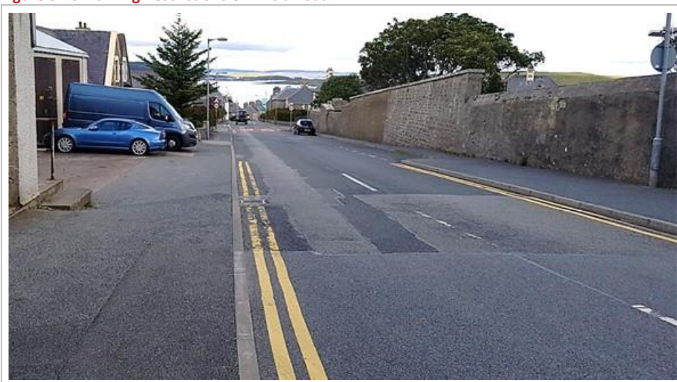
Figure 3.26 Parking Restrictions on Knab Road
