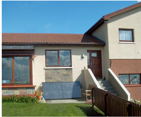
A solar thermal system installed in Sandwick
