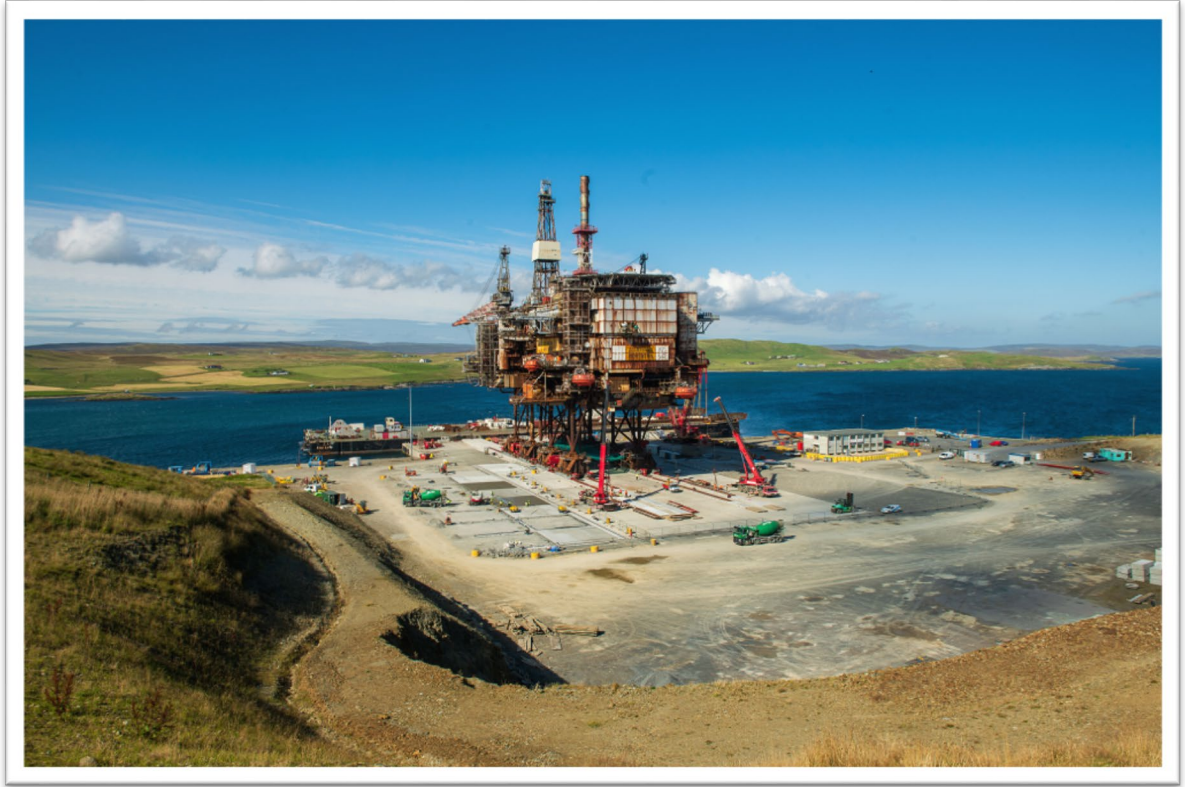
(Dales Voe decommissioning quay. Image: Lerwick Port Authority/Shetland Flyer Aerial Media)
