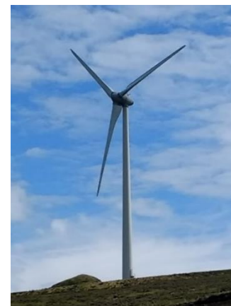
Figure 4 Luggies Knowe Wind turbine – original photo saved in Teams
